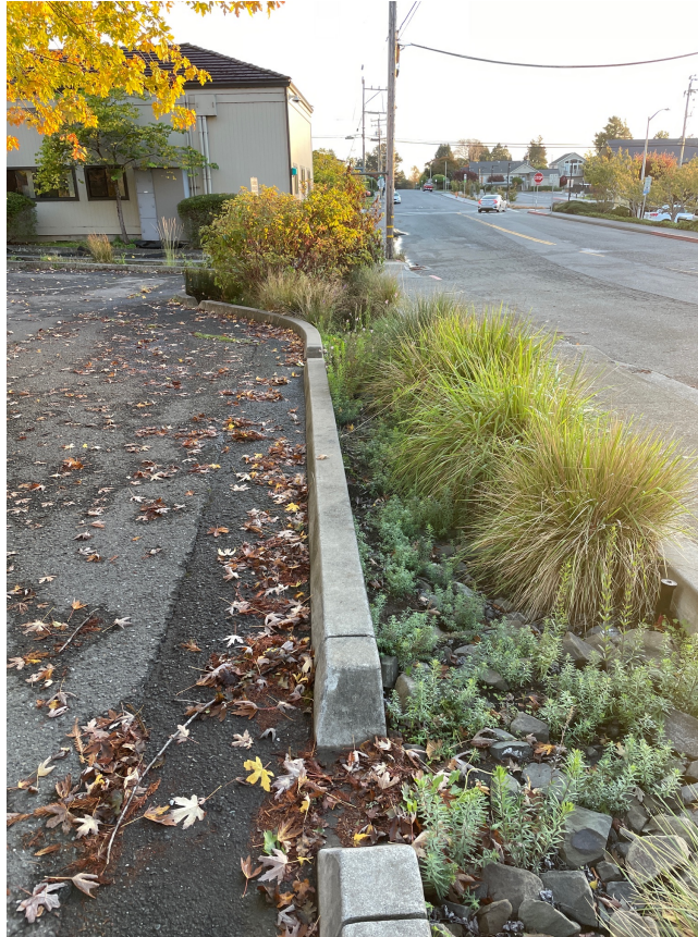
Figure 6. A bioswale at Cal Poly Humboldt allows parking lot runoff to percolate through vegetation and infiltrate into the soil rather than entering streams.
