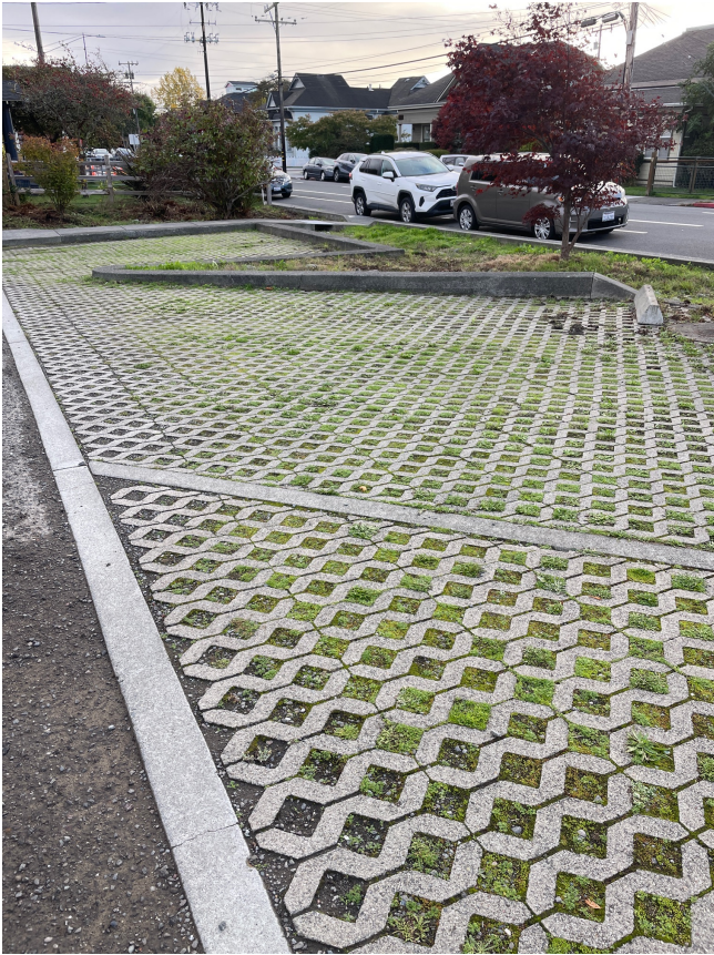
Figure 5. The City of Arcata's parking lot on 7 th and H Streets features permeable pavement and open pavers that prevent stormwater runoff from leaving the site.
